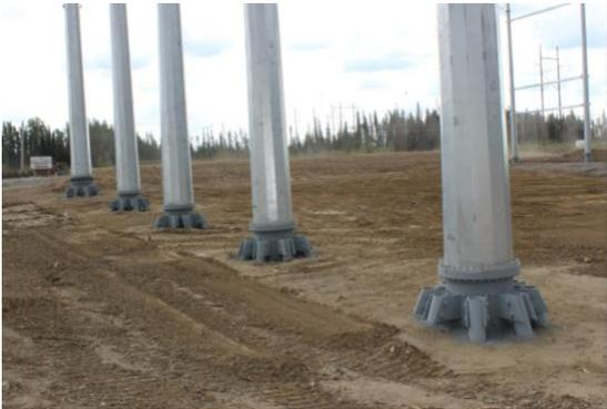
Grouted piles being installed to support large storage tanks:
