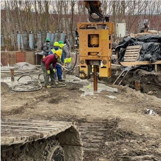
Bucket Pile for support of direct bury wooden poles:
