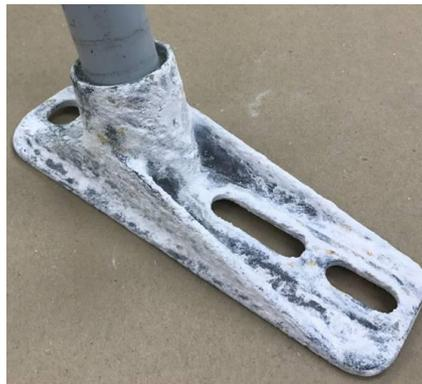
Figure 3 – Contamination Buildup on the End Fittings
